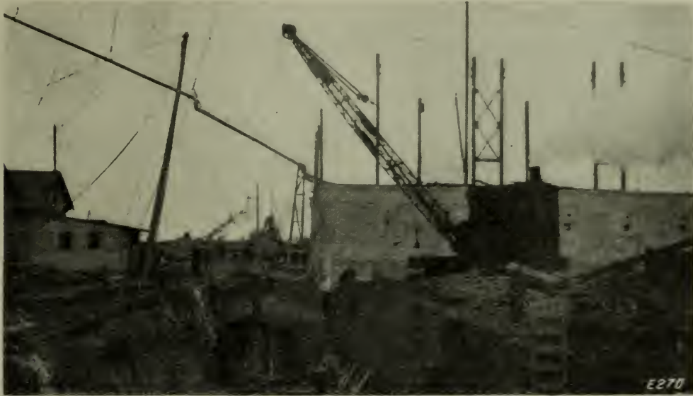
FIG. 11. STEAM SHOVEL AND LOCOMOTIVE CRANE.
